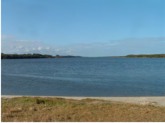
Photo 13. Northerly view from Lake Ponte Vedra dam
