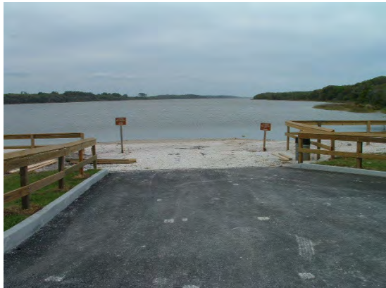
Photo 27. Boat ramp at Lk. Ponte Vedra dam
