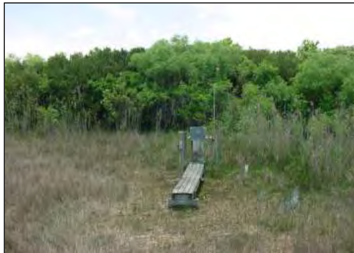
P34 Hydrological monitoring station.
